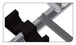
Arrange the backing plates so the 2nd plate overlaps and secures the 1st plate.
